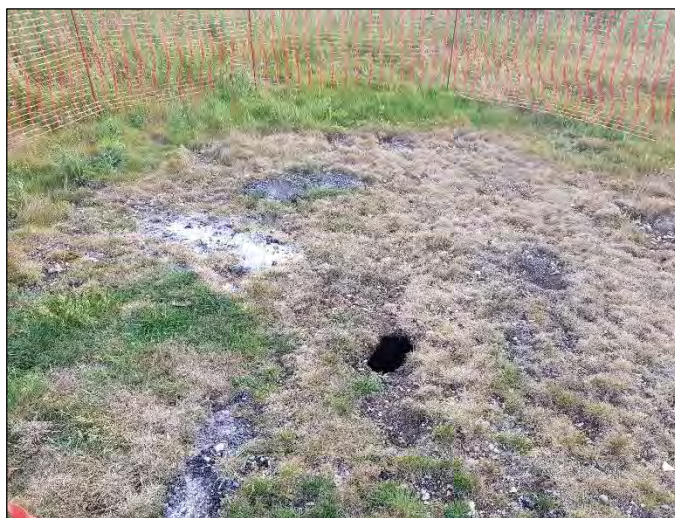
The latest sink hole - looks like it goes down forever...
