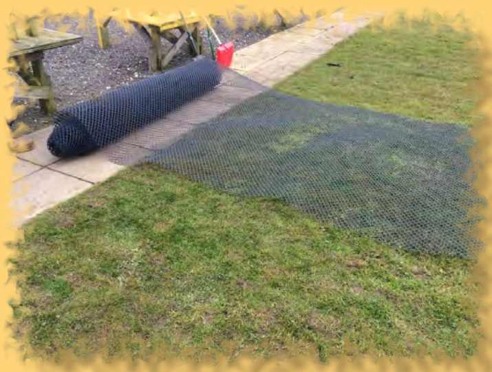
The start of the mesh laying process.
