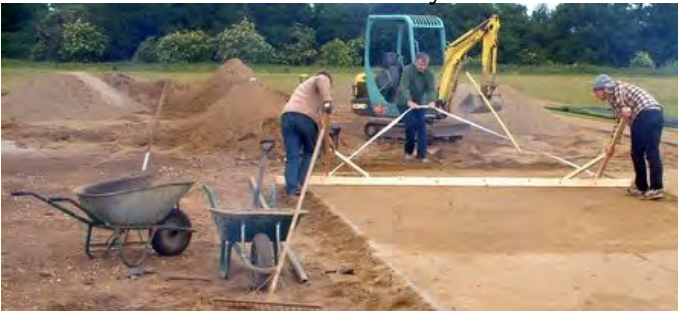
Above: The sand is spread and expertly "screeded" - levelled to provide a firm base for the new turf. Above right: At the school in Orpington, the Astro Turf hockey pitches are stripped and rolled for us.
