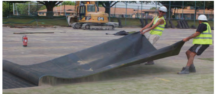
Above: The sand is spread and expertly "screeded" - levelled to provide a firm base for the new turf. Above right: At the school in Orpington, the Astro Turf hockey pitches are stripped and rolled for us.
