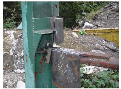
Repair completed by our Welder
