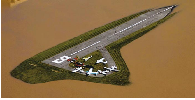
The West End of the Bloomsburg Airport runway became an island a few days ago in the flood-swollen waters of the Susquehanna River. Several planes and vehicles occupied the high spot yesterday as the owners waited for the high water to crest.
