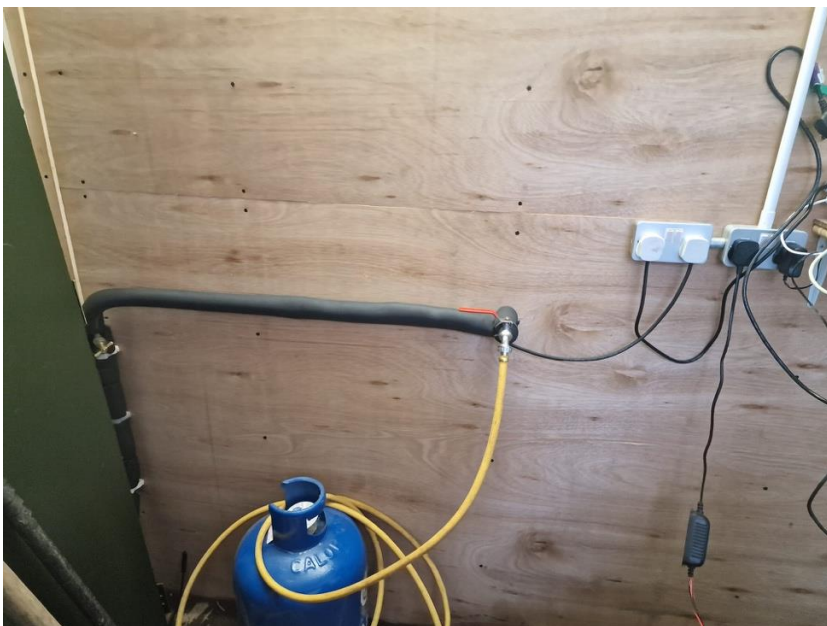
Water pipe work and new tap fitted.
