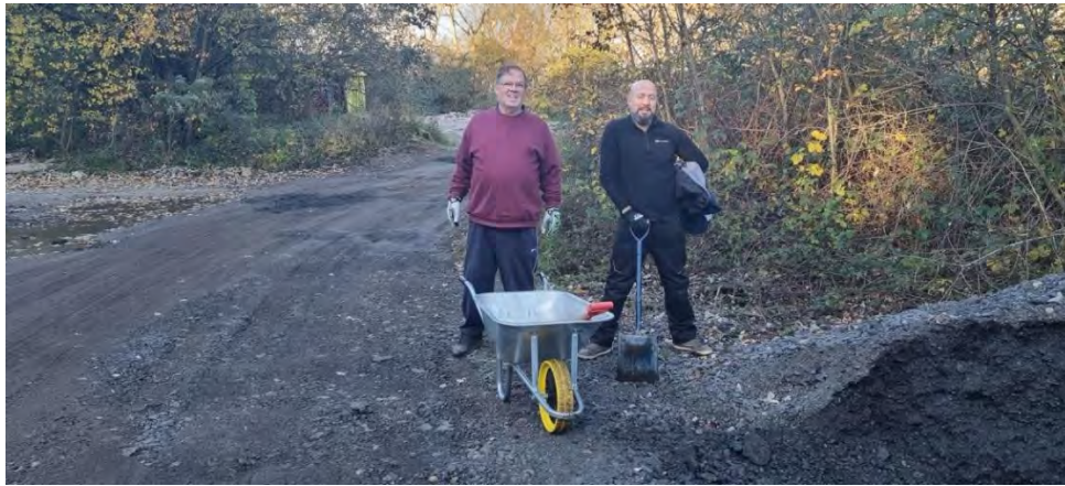
Pothole work party. Great job guys.
