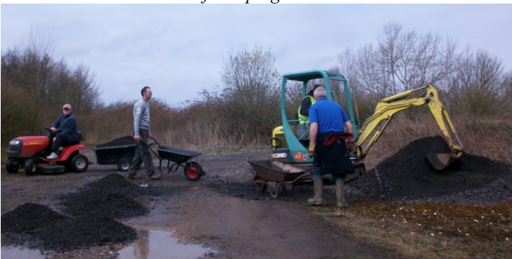
Filling more holes lower down the access road
