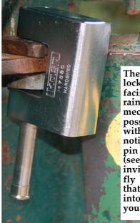
The gate padlock must be locked with the keyhole facing downwards to avoid getting into the nism. But it is rain mechanism. possible inadvertently to withdraw the key without noticing that the locking pin has dropped down, (see left) leaving an open invitation to vandals and fly tippers. Always check that the pin has clicked up into place before and after you withdraw the key.
